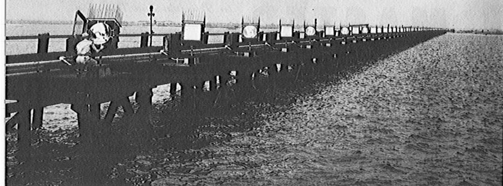
Photo credit The Port of New York Authority All Weather Landing Lights, N. Y. Airport
