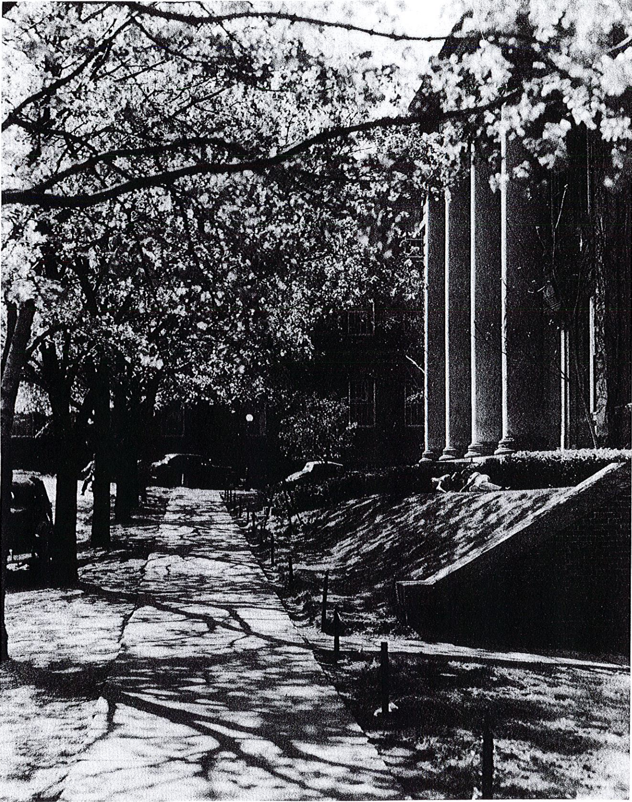
Troy Building, Rensselaer Polytechnic Institute Department of Civil Engineering and Department of Mechanics
