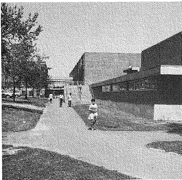
FIGURE 5. Engineering East - Part of the new Engineering Complex.
