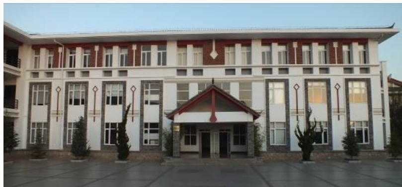
Figure 4. The Actual Photograph of Wen-Zhi Building(1:150).
